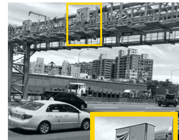
An ETC system employed on highways in Taiwan. Just pass through the sensor installed above the road to pay your toll. This innovation has made manned toll gates unnecessary in Taiwan. → p. 66
