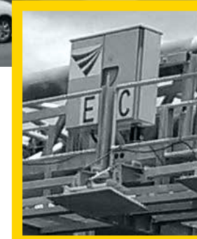
An ETC system employed on highways in Taiwan. Just pass through the sensor installed above the road to pay your toll. This innovation has made manned toll gates unnecessary in Taiwan. → p. 66
